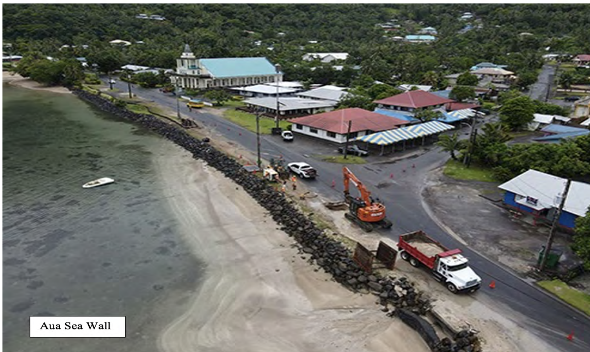
Aua Rockwall Revetment Photo Courtesy DPW
